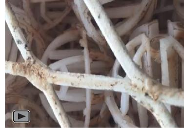
(c) *Bottom Support Grid:* Support grid appears clean and free of calcification and scaling.
